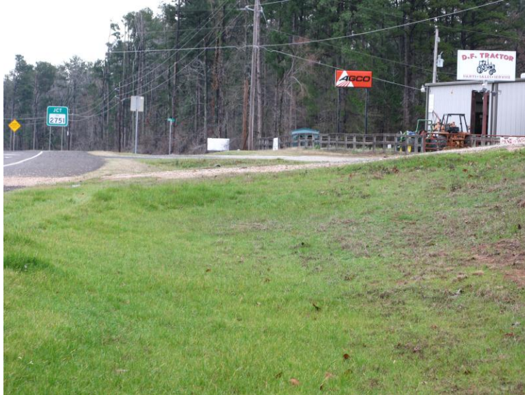
Looking south from easement centerline, that gravel drive is the current access point from hwy 259, there is no drainage there and water pools
